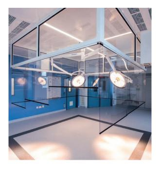
The MAT body exhaust system chosen by Royal Hallamshire Hospital offers another layer of protection for patients and users. Tests have indicated that when used in conjunction with the MAT ECO-flow™ UCV canopy, the number of Bacteria Carrying Particles or Colony Forming Units can be significantly reduced.
