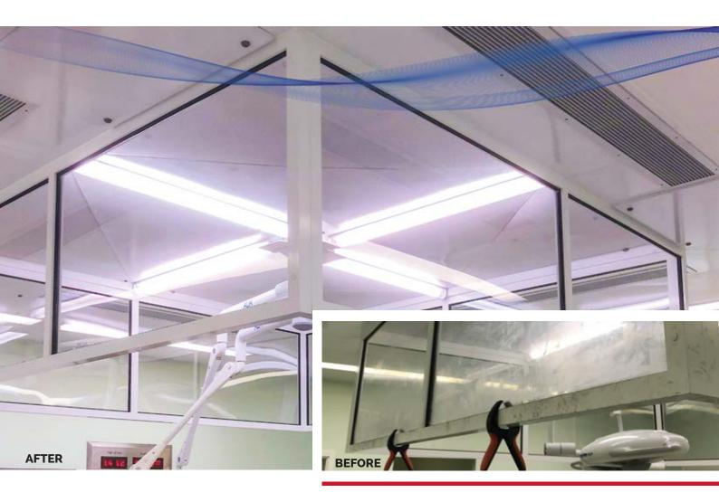
Over time, the glazed polycarbonate panels around the perimeter of an ultraclean ventilation (UCV) canopy can become scratched and damaged and the paint finish on the aluminium frame can flake. This not only makes the operating theatre look tired but can also cause issues around infection prevention as chips and scratches can harbour dangerous bacteria.
